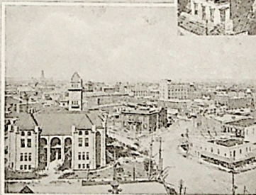
VIEW FROM POST OFFICE-NORTH EAST
